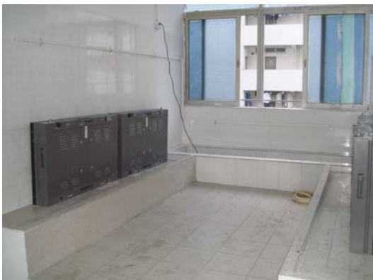
Splitting Water-proof Test
