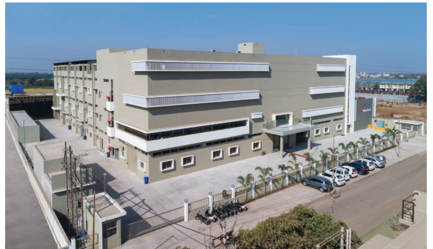
Unit 2 | 2400 Metric Ton / Annum Handling Medium to Large volume Inhouse Machining & Assembly
