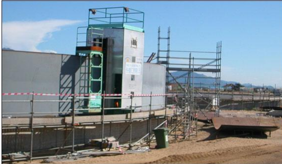
All Time EGW used for tank erection
