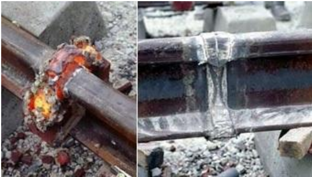
Photos of Thermit Welding Process
