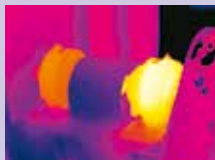
Overheating bearing cap
